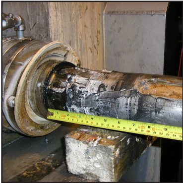
View of worn bearing seat area on shaft
