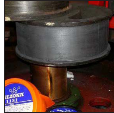
Another close up of the repair
