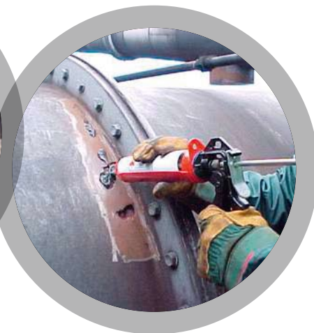
Infill of Corrosion Pits
