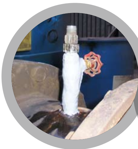
Leak Sealing of Pipework
