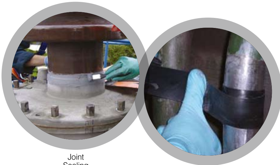
Oil Leak Repair
